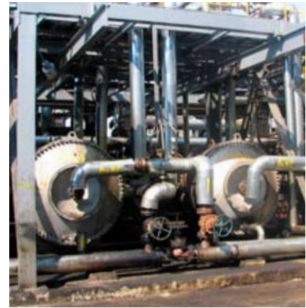
Two of the eight spiral heat exchangers.
