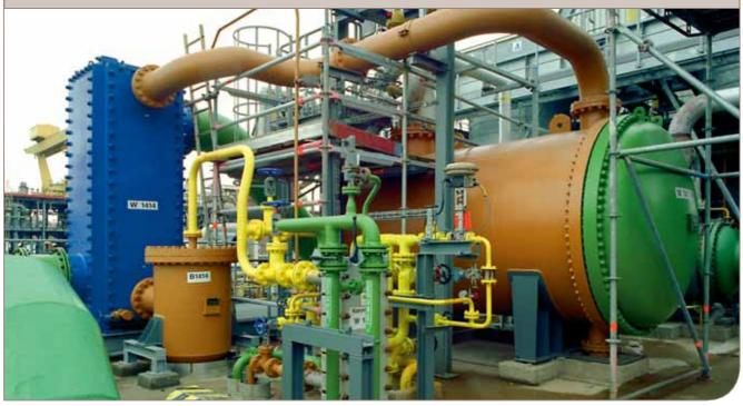
The Compabloc and the shell-and-tube units are installed in series. The Compabloc has a higher heat load, and allows for both condensation and sub-cooling, but is much smaller in size.
