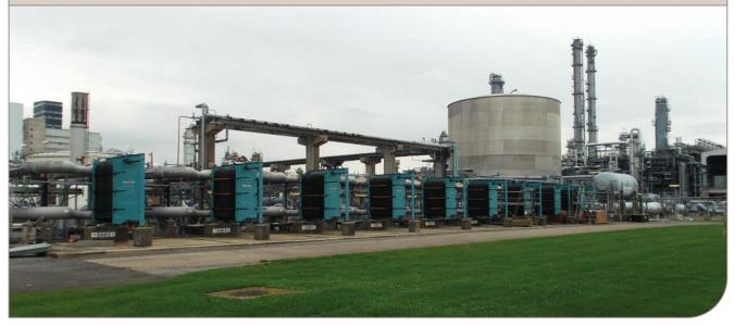
Nine Alfa Laval M30 units are responsible for cooling down the process water of the steam cracker.
